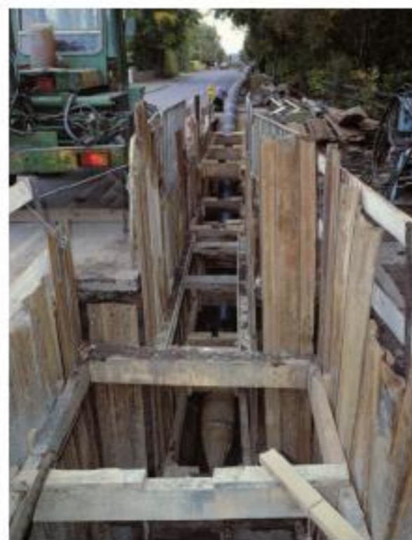
▲ An earthwork support prevents the trench from collapsing
