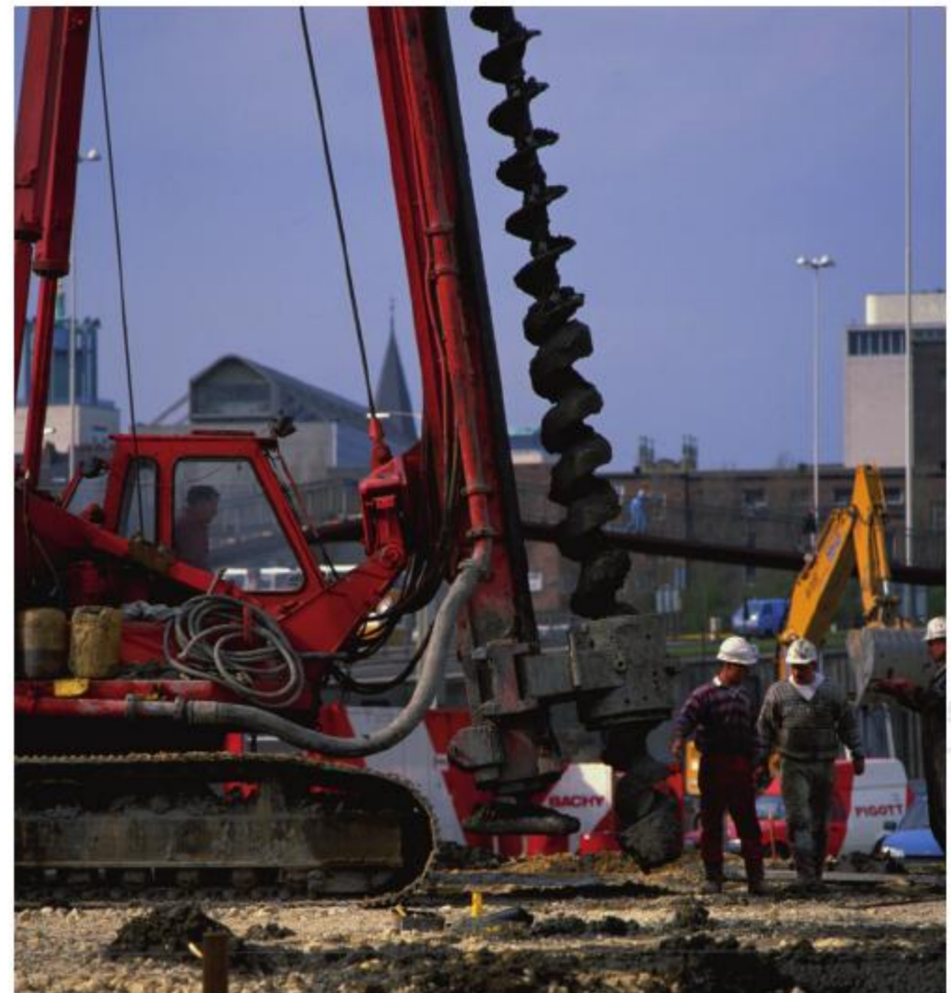
▲ A piling rig with auger drill
