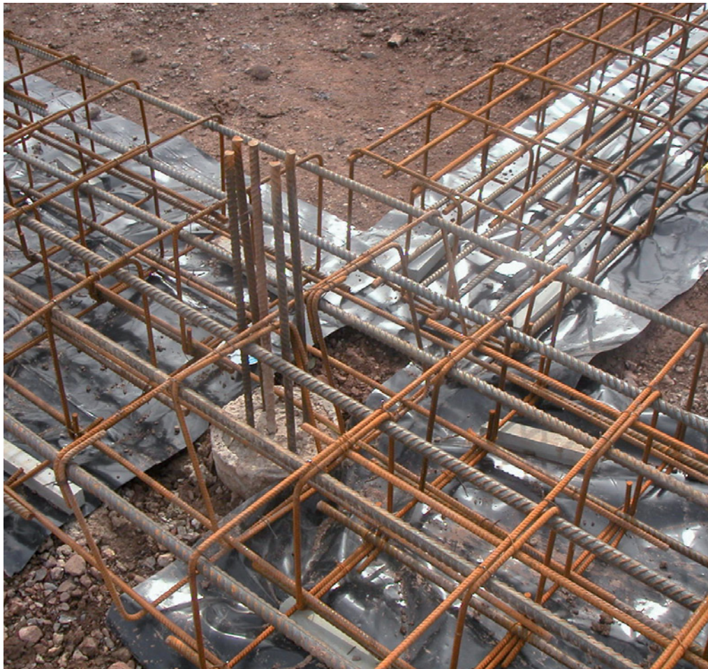
Figure 16 Pile and ground beam reinforcement.
