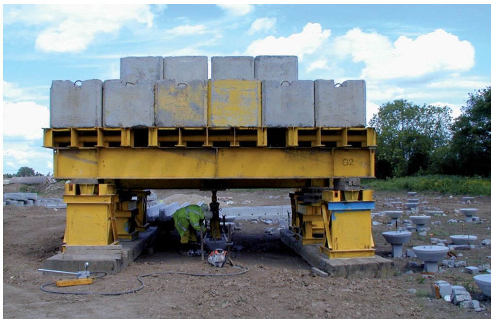
Figure 26 Static load testing of piles using kentledge.
