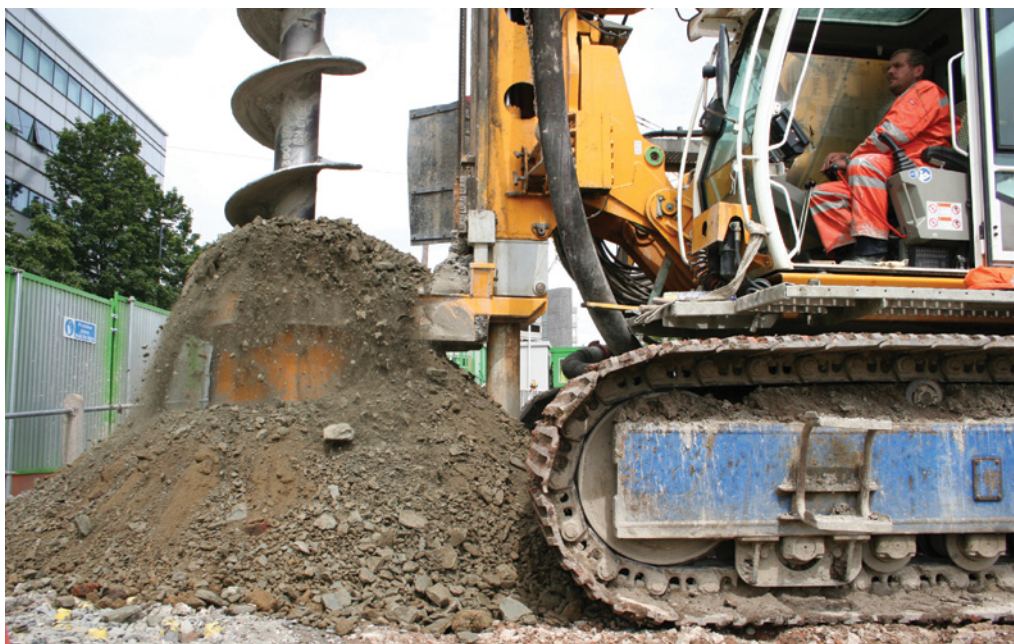
Figure 21 Continuous flight auger bored piling.
