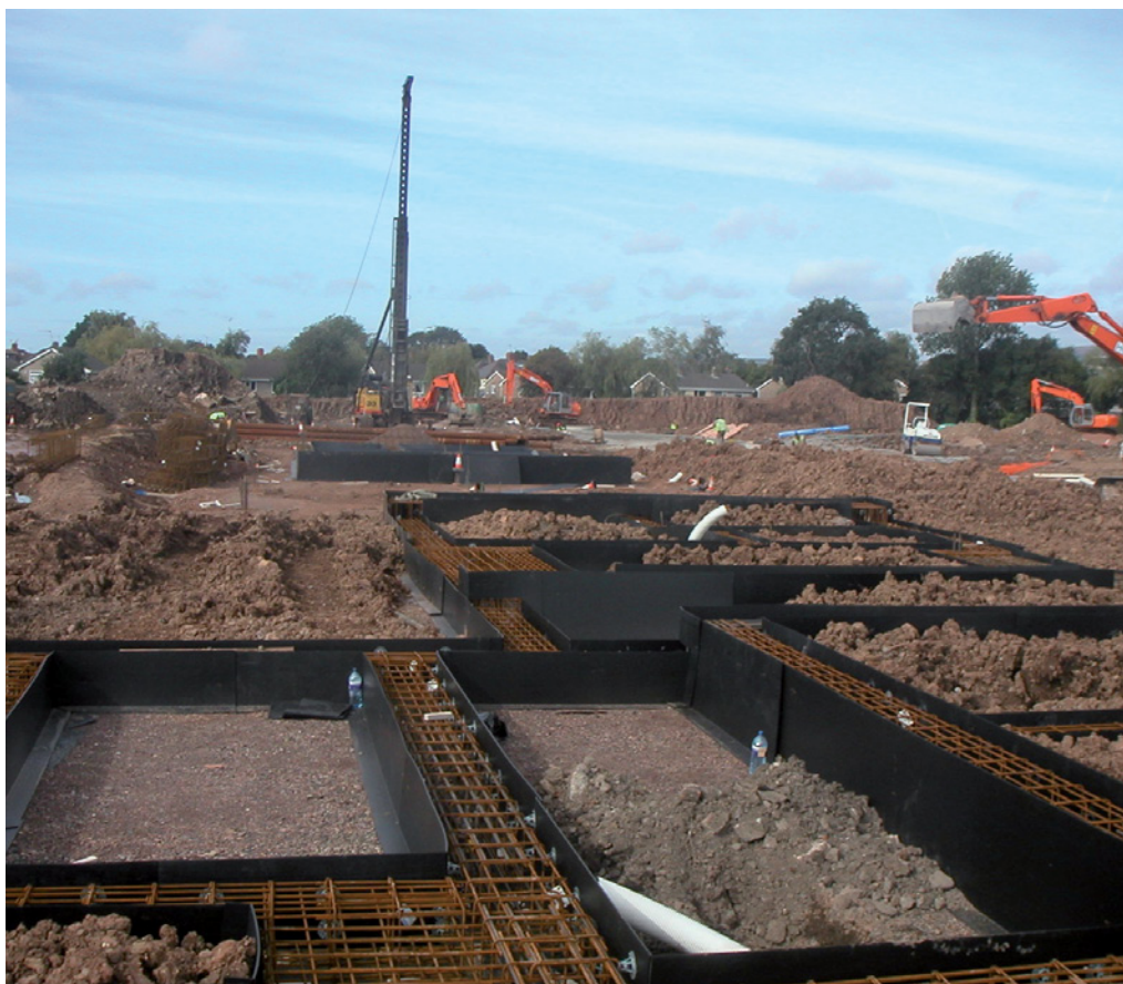
Figure 17 Ground beams prior to casting of concrete.
