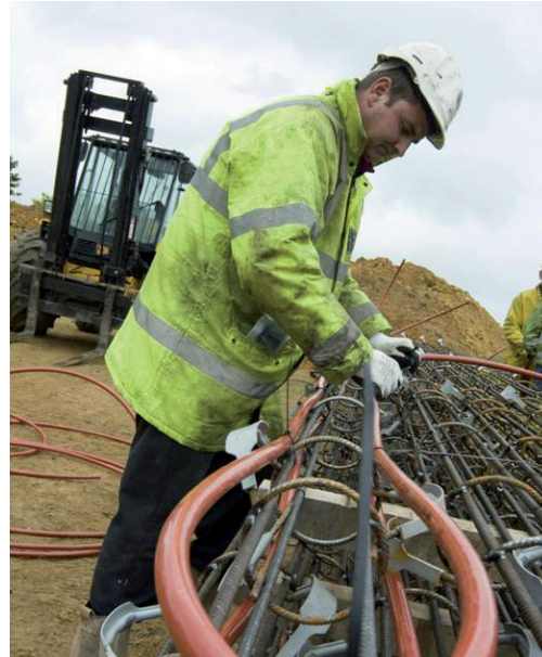
Figure K1 HDPE pipework being fitted to the reinforcement cage for a pile.
