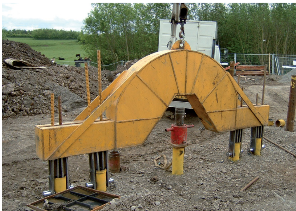
Figure H2 Static load testing using reaction piles.
