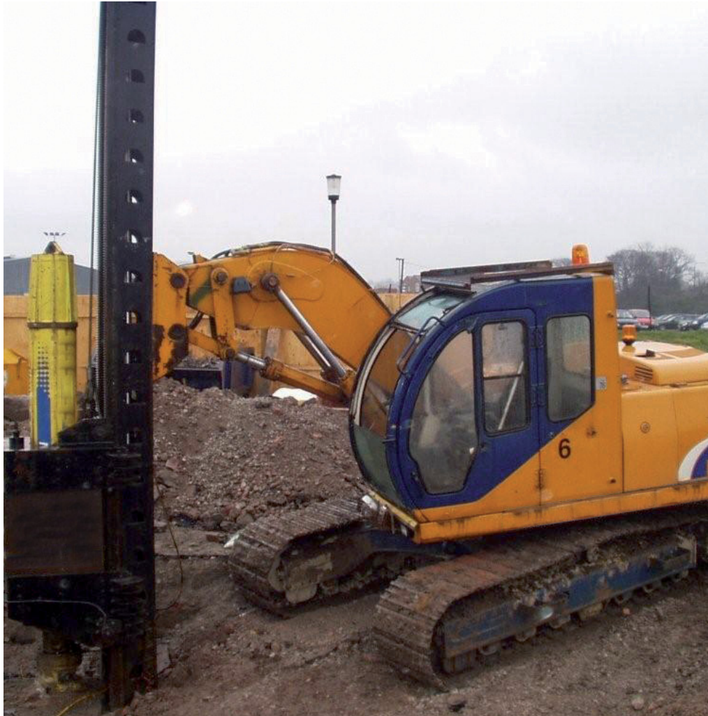
Figure H3 Example of a crawler mounted 1 MN statnamic test system.
