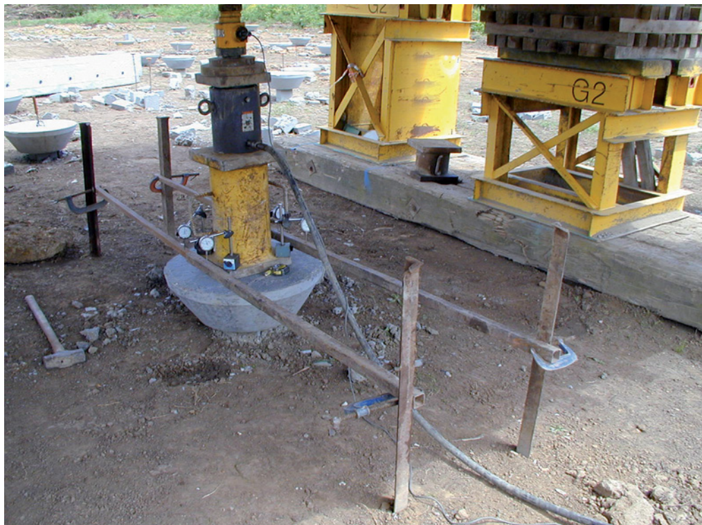
Figure H1 Static load testing of piles.
