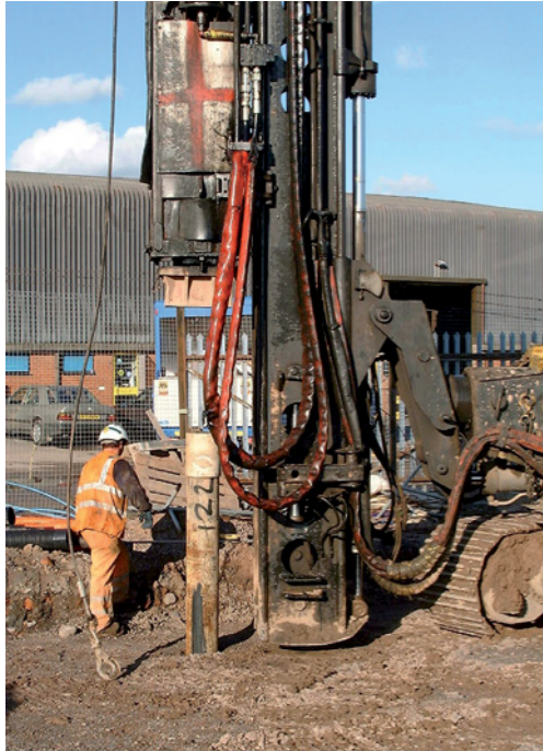
Figure 19 Installation of driven steel piles.
