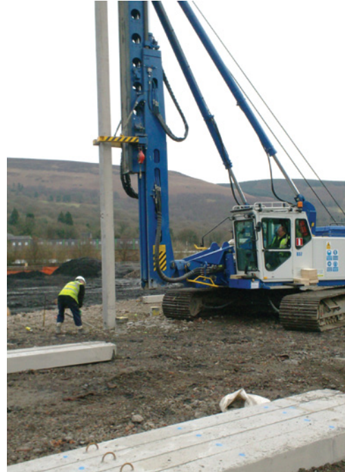
Figure 20 Installation of driven pre-cast concrete piles.
