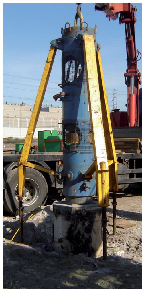
Figure 27 Dynamic load testing of piles (Image courtesy of PMC pile testing).
