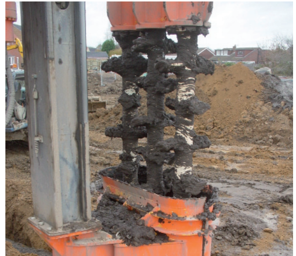
Figure 12: Triple auger soil mixing system
