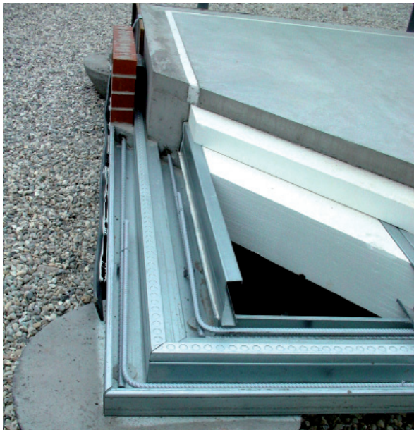
Figure 7: Proprietary foundation system comprising insulated ground floor slab and reinforced concrete perimeter beam, supported on piles
