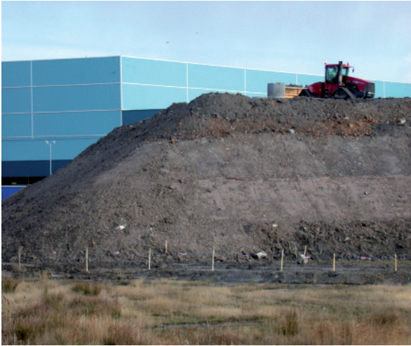
Figure 3: Surcharging fill to reduce the risk of collapse compression
