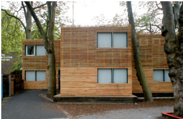
Figure 10: Modular buildings supported on screw piles, near to trees
