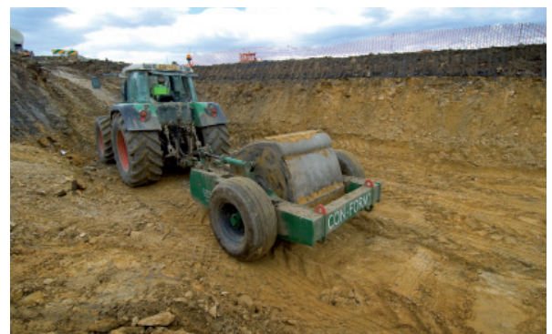
Figure 13: Roller dynamic compaction
