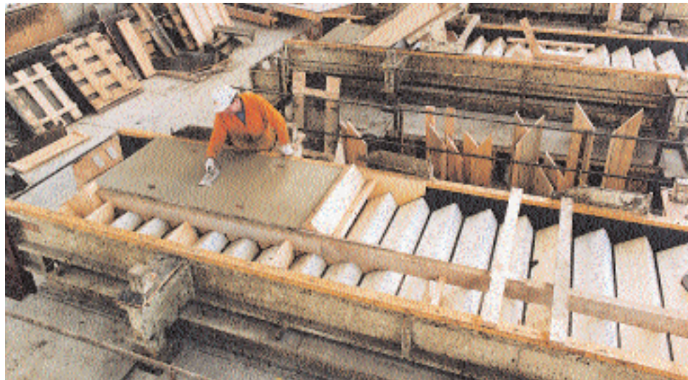
Off-site production of staircase components (courtesy of Tarmac Topfloor Ltd)
