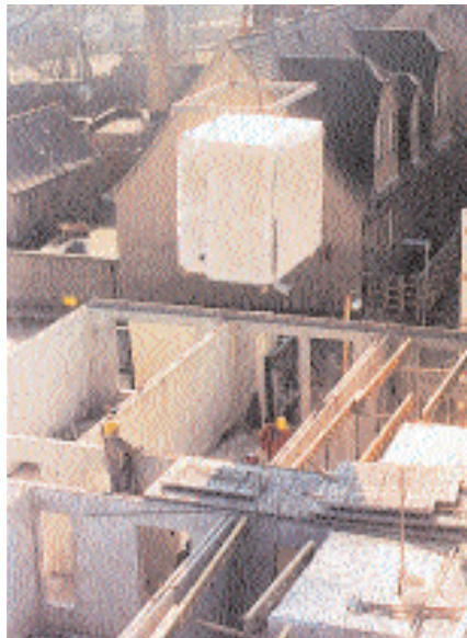
Installation of bathroom pod (courtesy of PlanTech Badsysteme GmbH)
