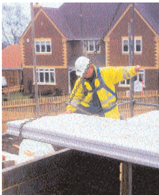
The preferred solution: Traditional construction and high performance hollowcore (courtesy of Bison Concrete Products Ltd)
