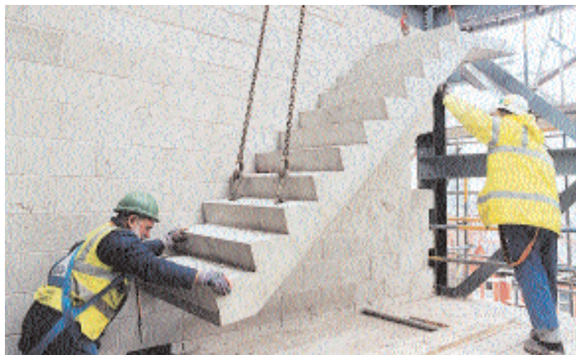
Components: Placing a precast concrete staircase, (courtesy of Tarmac Topfloor Ltd)
