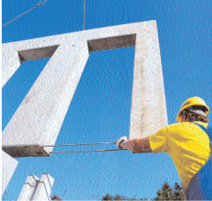
Precast concrete contributes to on-site efficiency (courtesy of Veit Dennert KG)
