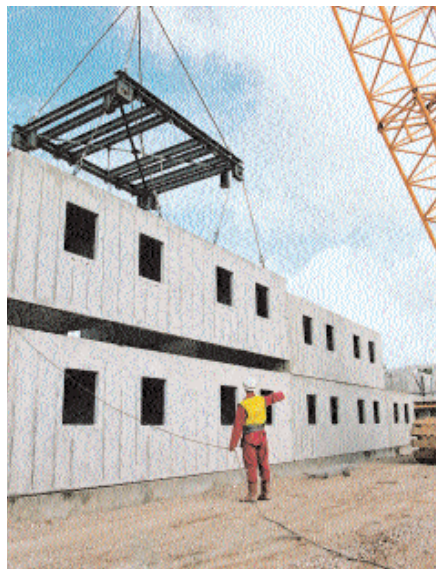
Left: Twin-room precast modules (courtesy of Tarmac Precast Concrete Ltd)
