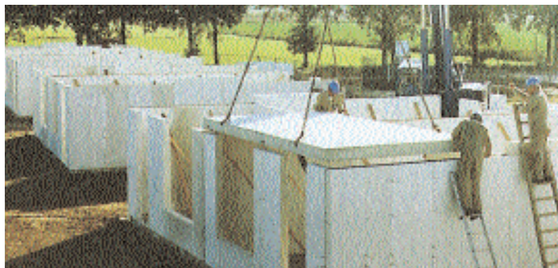
Speed of erection on site (courtesy of Belton/Bevlon)
