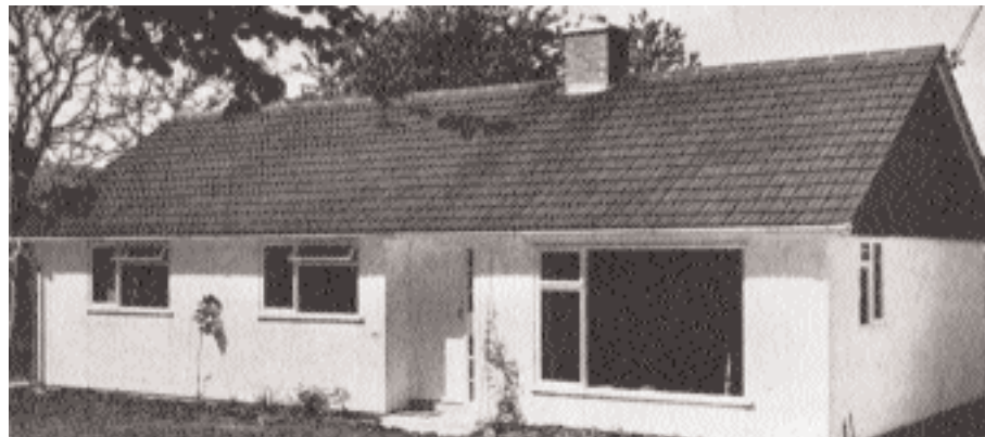
Past precast: The 'Woolaway' bungalow UK, circa 1960
