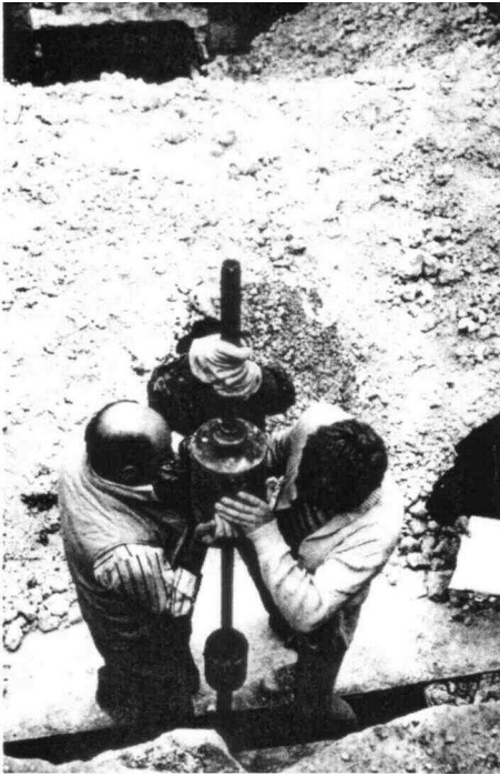
Figure 2.5 Using the standard penetration test equipment in chalk at a property development site in Leatherhead, Surrey.
