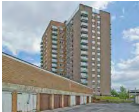
Council estates fast became the accommodation of last resort, as families on middle incomes sold up and moved out
