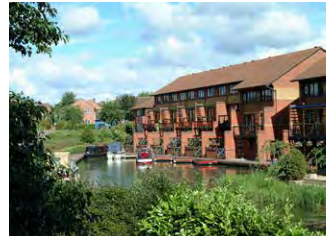
Pennylands in Milton Keynes, a large-scale pioneering project exploring passive solar design
