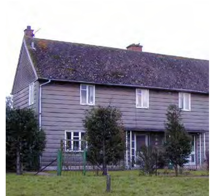
Surviving Airey houses clad in their hallmark precast concrete panels. In 10 years from 1945 to 1955 over 26,000 were built in England and Wales
