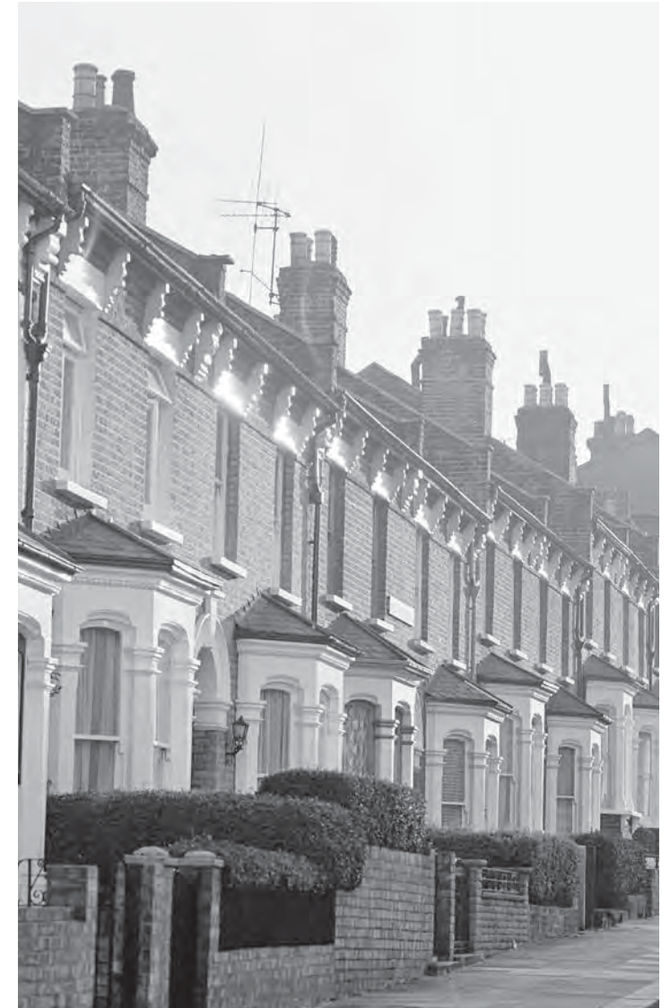
Elegant exteriors and a chimney-dominated skyline along Northwood Road, London. An illustration of the popular perception of Victorian housing
