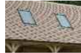
Rooflights Conservation rooflights offer an alternative to the dormer window and are often preferred by Local Authorities.
