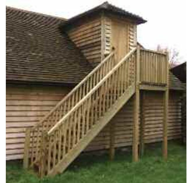
External Oak Staircase 900mm wide open treads. Handrail 100 x 75mm, newel posts 125 x 125mm
