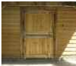
Stable doors Standard sizes: Equestrian - 1.25m wide x 2.1m high Domestic - 0.9m wide x 2.1m high
