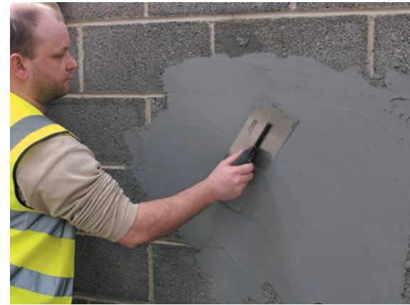
Plaster being applied and trowelled
