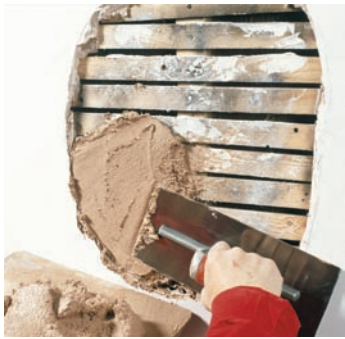
Lath and plaster
