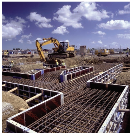
All buildings have a substructure
