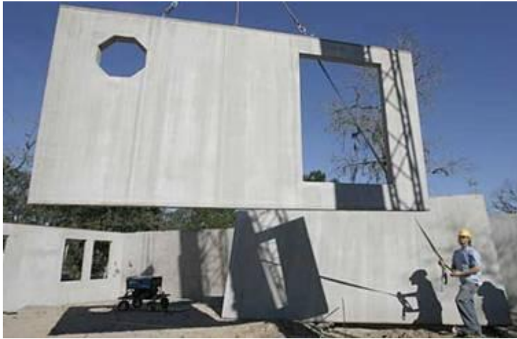
Precast Concrete & SIP's Panels
