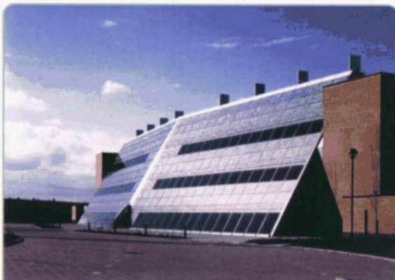
Doxford Solar Office, Sunderland
