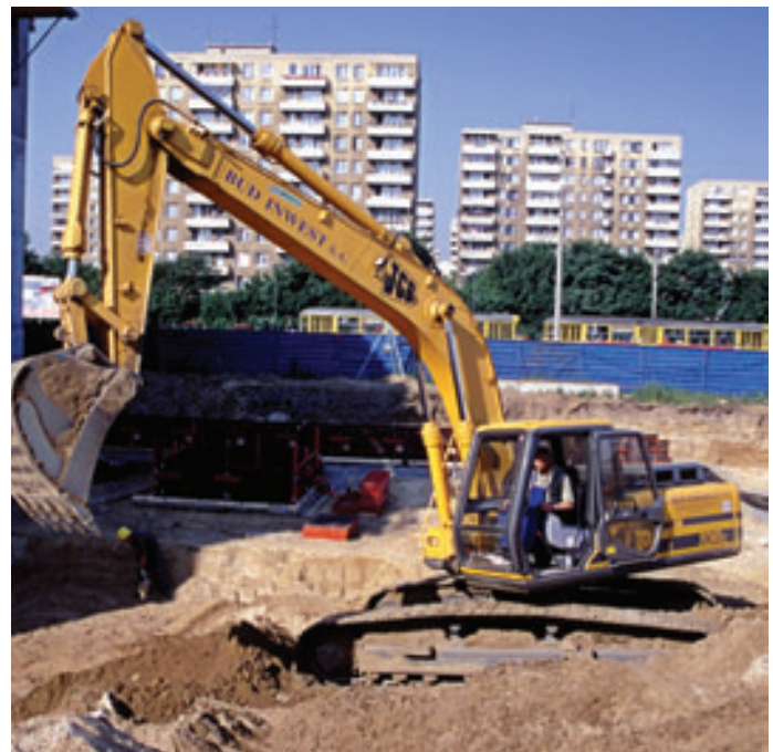
Removing soil from a site
