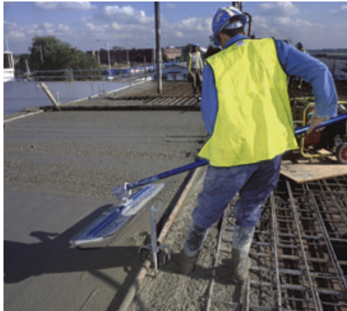
Steel reinforcement of concrete
