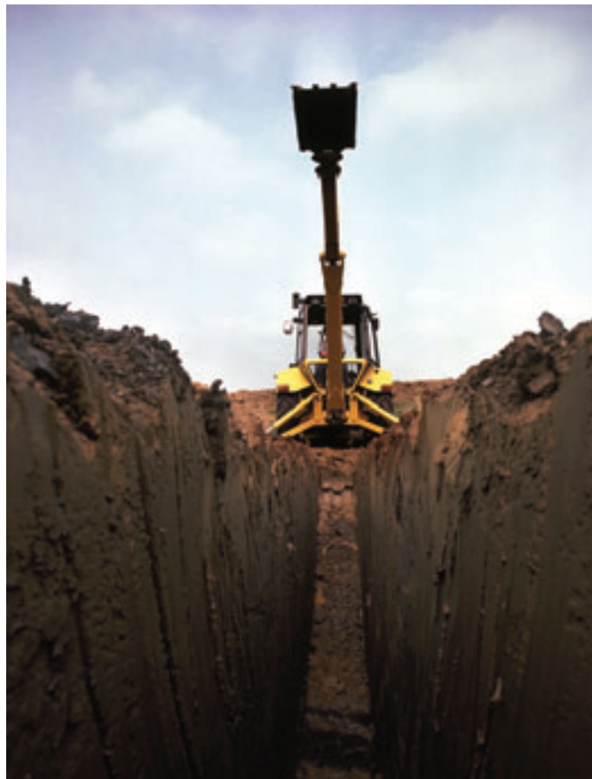
Trenches are often excavated by mechanical means
