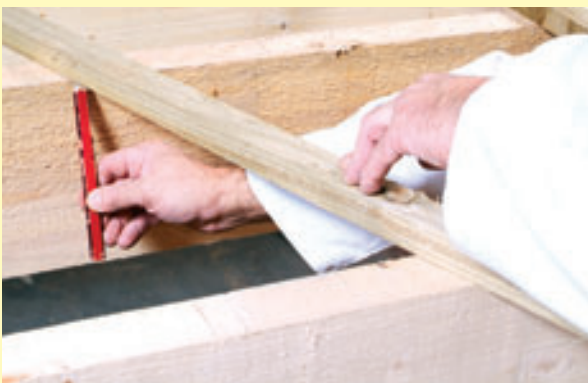
Lay struts across two joists at a diagonal
