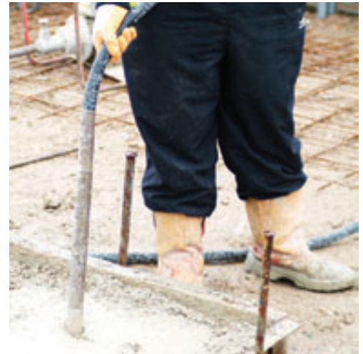
Vibrating poker in use
