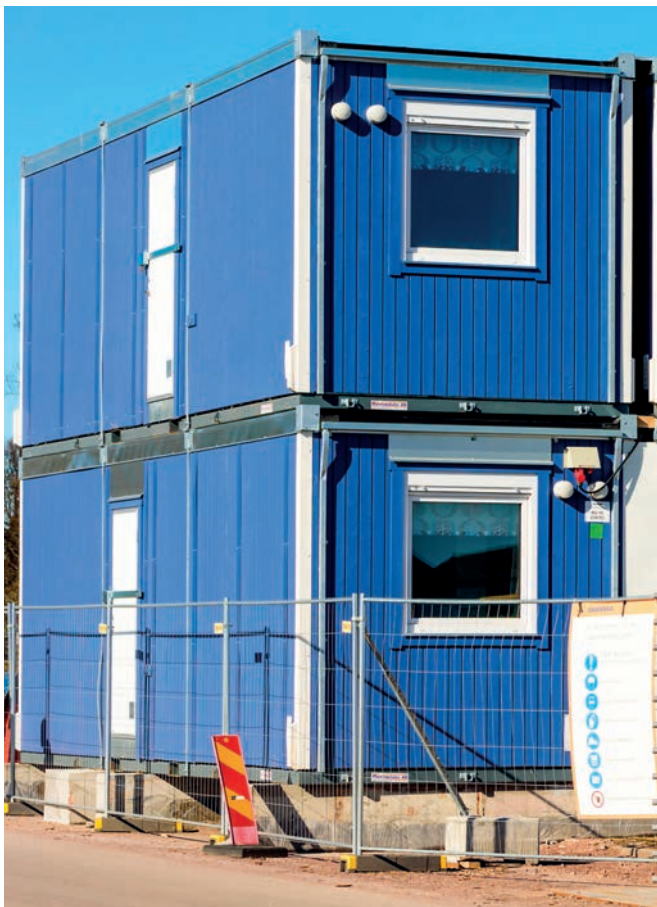
► Piggybacked site storage cabins save space
