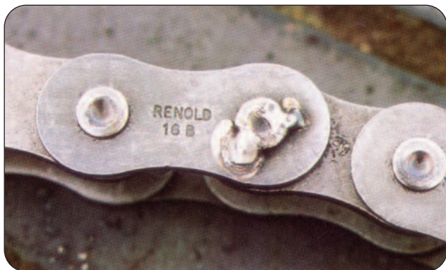
Figure 6 - Mode of Failure - Cracking
