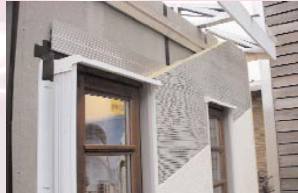
External wall insulation applied to a steel-framed building
