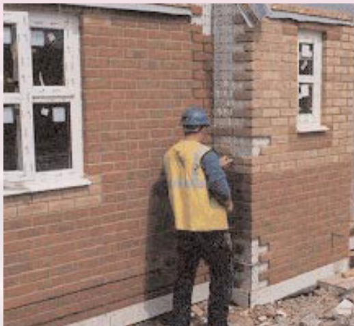
Brick Slips fixed to steel framed building
