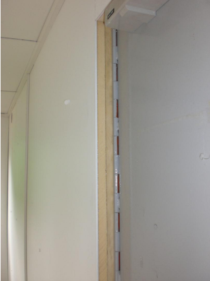
Photo: Insulated plasterboard installed (Courtesy of UKCG)
