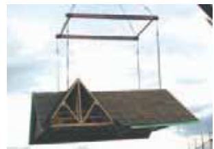
Pre-assembled roof structure being lifted into place
