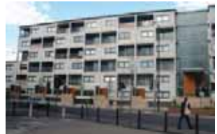
Completed block of flats in volumetric construction
