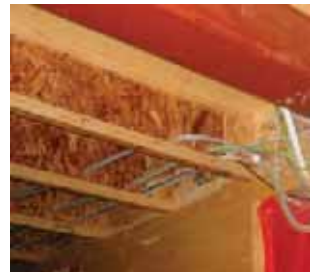
I beam timber joists
