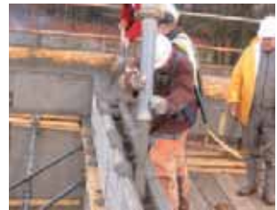
Concrete being poured into insulating formwork
