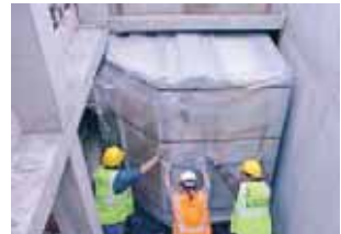
Pod being placed within a structure
