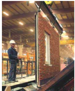
Concrete panels complete with insulation and half brick cladding
