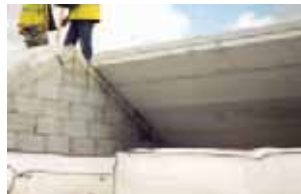
Aircrete planks used to create a roof deck
