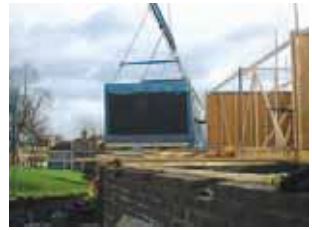
Volumetric unit being placed alongside panels
