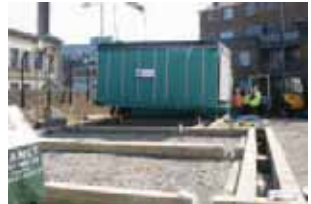
Volumetric unit being placed on levelled substructure
