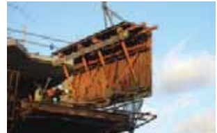
Figure 4 Steel shutter being removed from tunnelform after casting a bay
