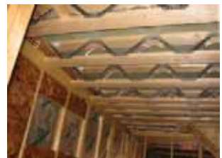
Metal web joists
