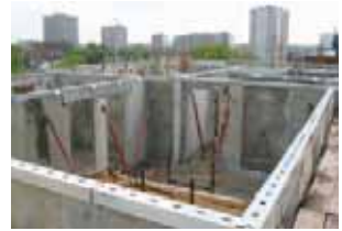
Composite panels being used to construct a block of flats
