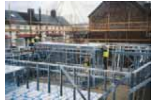
Steel framed floor cassette being lowered into place
