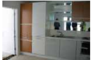
Volumetric unit as delivered to site showing level of internal fit out
