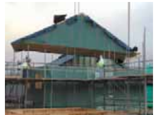
Roof cassettes being installed
