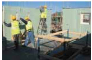
Closed timber frame panels being placed
