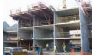
Figure 2 Tunnelform construction
