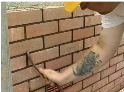
Bricklayer finishing joints with a bucket handle – a quick and effective joint.
