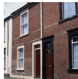
This bond is known as Flemish bond. It's common in houses built before the 1920s. The headers bind the two halves of the wall together. These walls are normally 215mm (1 brick) thick.
