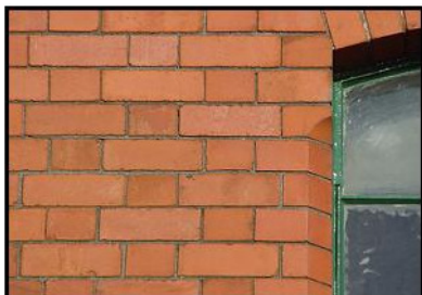
This bond is known as Flemish bond. It's common in houses built before the 1920s. The headers bind the two halves of the wall together. These walls are normally 215mm (1 brick) thick.
