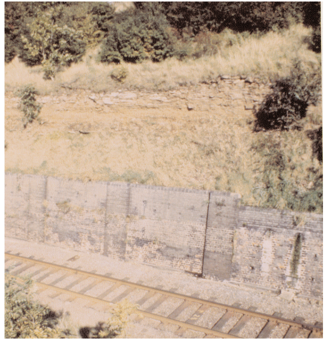
Fig 7 Soil and rock... 'exposure of soils or rocks in railway cuttings'
